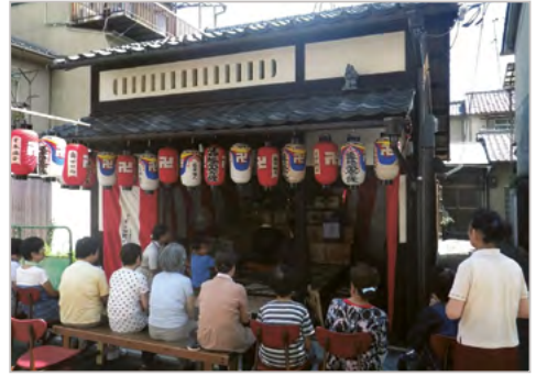
The small Saimoto Machiya in Kyoto is a house that is too small for a separate shop, therefore a combined working- and living space is situated towards the plinth. On ceremonial days the façade of the plinth will be removed and a neighbourhood temple or a place for children to play can be created, outside and inside becomes one space.
