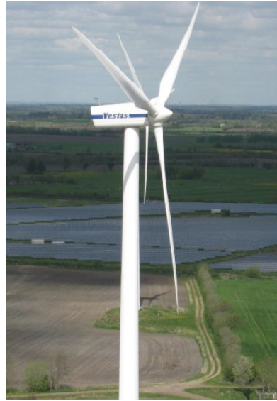
Fig. 3. The Vestas V66 wind turbine under measurement.
