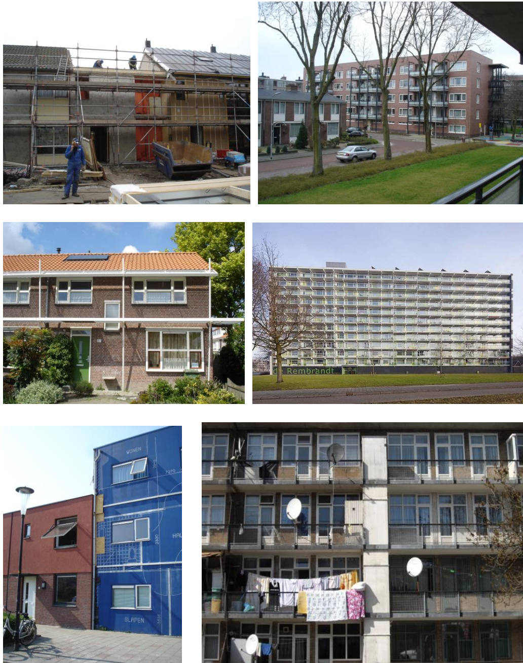
Figure 3: Impression of the six renovation projects.
