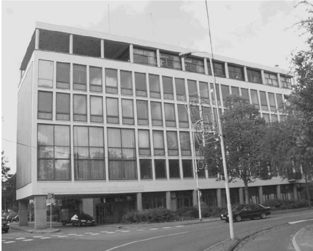
Figure 4. Existing office building.
