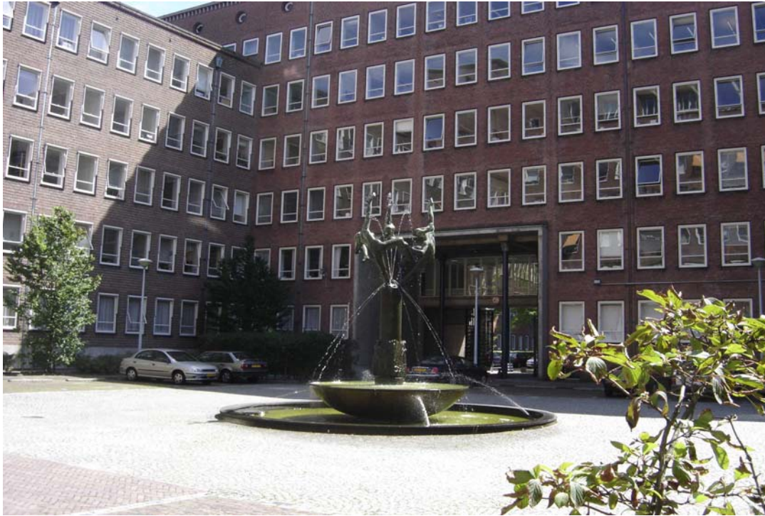
Figure 3 - Exterior of the Ministry of Agriculture building
