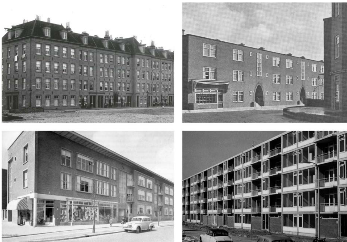
Figure 3: Four subtypes tenement apartment blocks; left above subtype 1 inter war Amsterdam, left right subtype 2 inter war Den Haag, left below, subtype 3 post war mix traditional and construction system, right below subtype 4 post war dry prefabricated construction system
