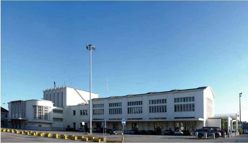
Fig. 3 Alcântara passenger terminal, 2007. The building hosts today the headquarters of the APL. Author: José M. P. Sánchez; released under a Creative Commons Attribution-NonCommercial-NoDerivatives 4.0 International License
