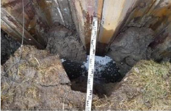
Figure 16. Gapping behind sheet pile wall AZ26
