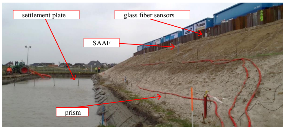
Figure 7: Monitoring campaign FST on (non-)reinforced test levee
