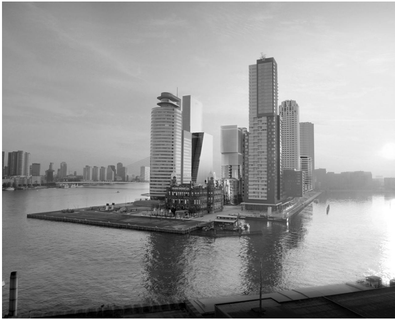
Figure 3.7 Wilhelminapier/Kop van Zuid (Source: Municipality of Rotterdam, 2010)
