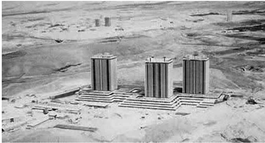
FIG. 3.13 ASP residential complex in the west of Tehran. / Source: Art and Architecture , number 47-48.
