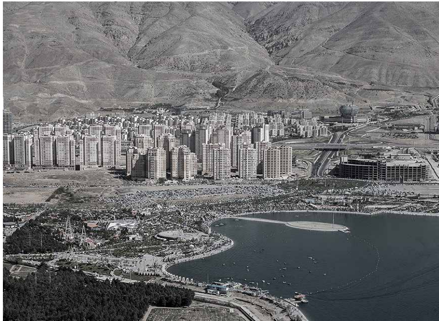
FIG. 6.11 The excessive construction of dispersed high-rises in District 22. / Source: Mohsen Ataei.
