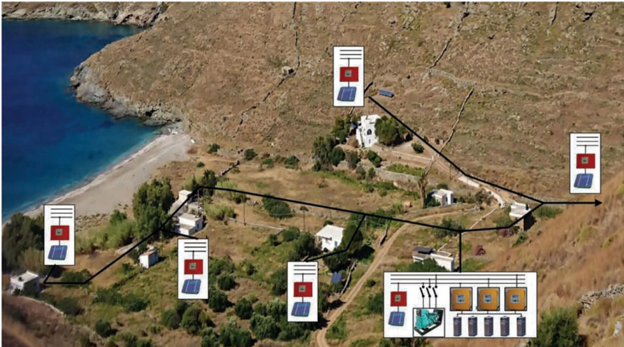
Figure 13. Overview of Gaidouromantra Microgrid in Kythnos island.
