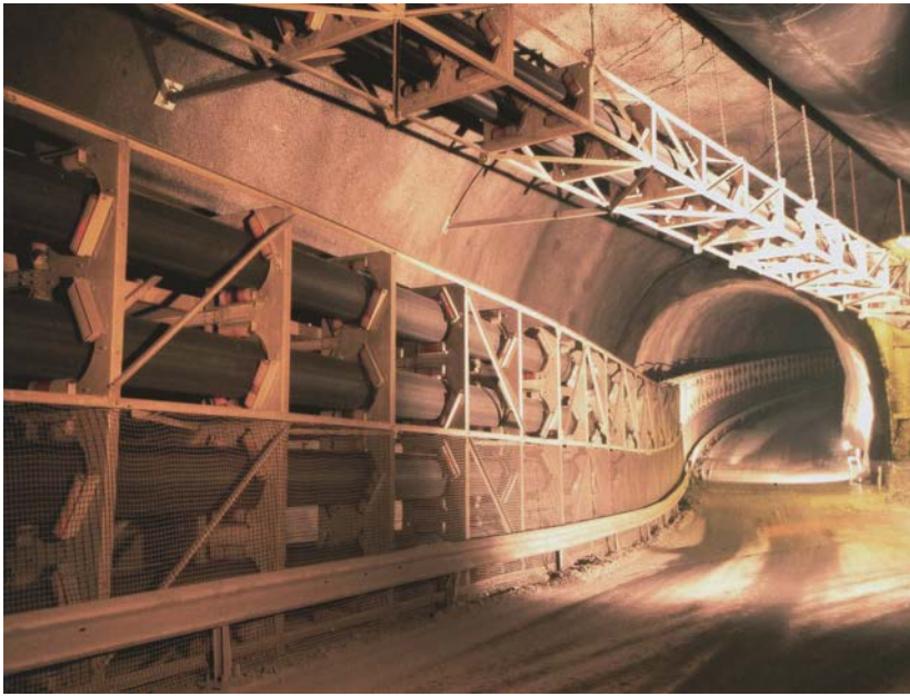
Figure 1.4: Pipe conveyors transporting bulk solids through a narrow tunnel passage during the construction of Lötschberg base tunnel in Switzerland (Image courtesy FLSmidth Wadgassen GmbH).
