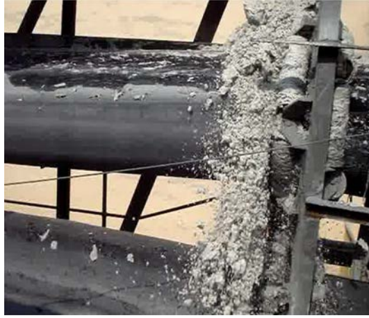
Figure 2.5: Overloaded pipe conveyor in Kailin, Guizhou Province, China (Image courtesy Dr. Robin Steven).
