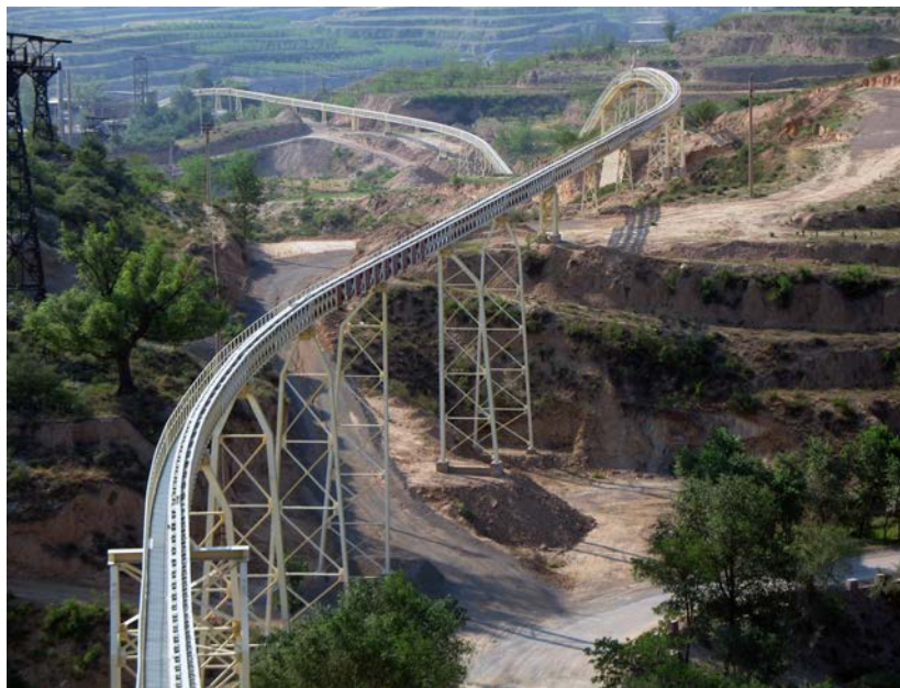
Figure 1.3: Pipe conveyor operating in complex topographical conditions in Taiyuan, Shanxi Province, China. The route passes over the rocky terrain, mountains, farms, roads and small communities (Image courtesy FLSmidth Wadgassen GmbH).
