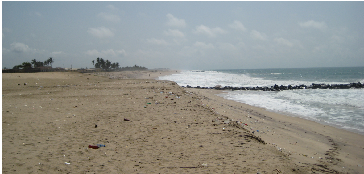
Figure 2-4: The Ada sea defence project, at Ada Foah, looking East. On the left the nourished beach barrier and to the right a groyne. The step in the coastline is an effect of the groyne partially blocking the sand.
