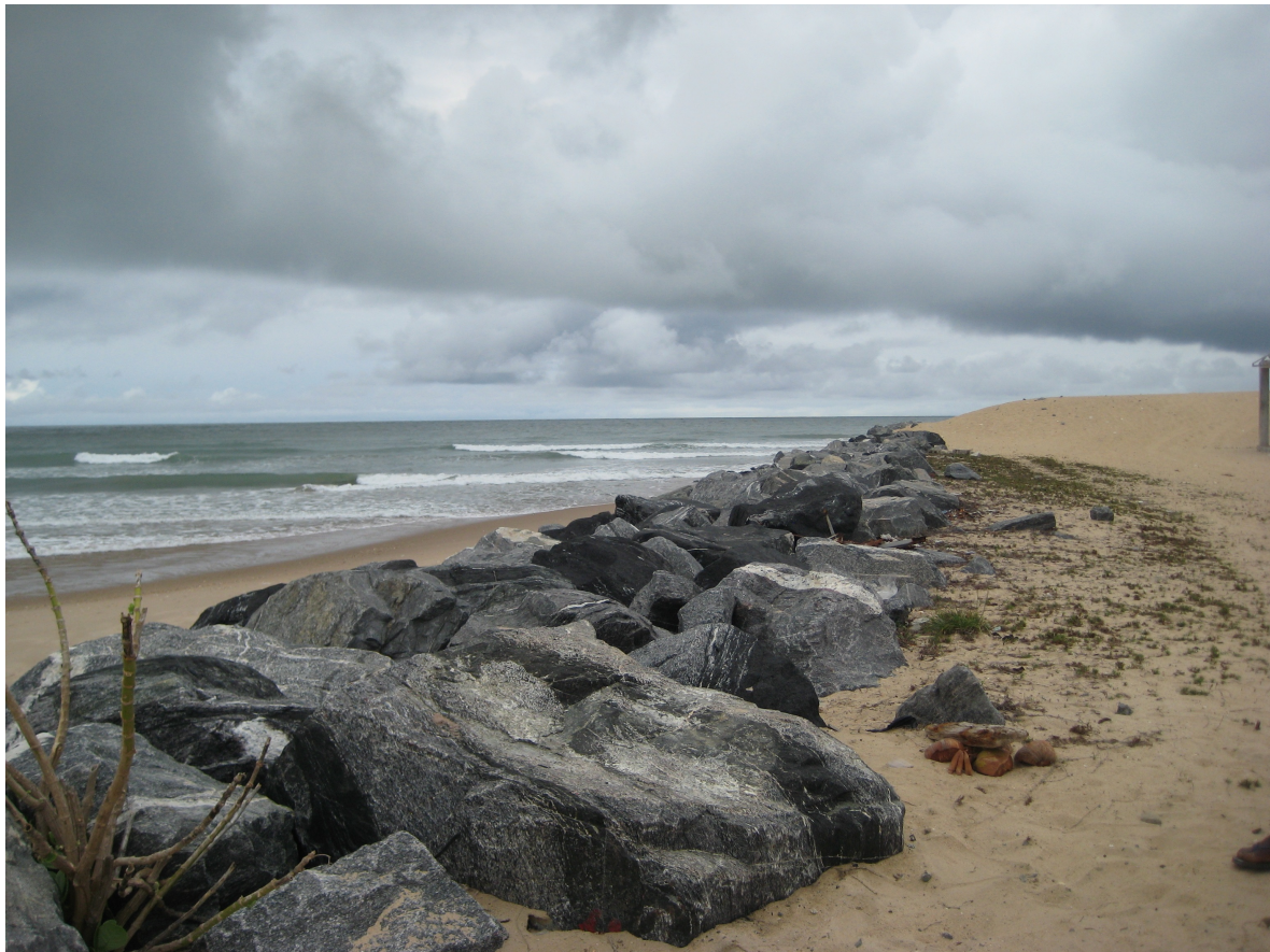
Figure 2-5: The Ada sea defence project, at Kewunor, looking south. Visible is the last groyne west of the Volta river mouth (to the left) and the beach barrier to the right. The spit used to extend across the river mouth, but has largely been eroded.
