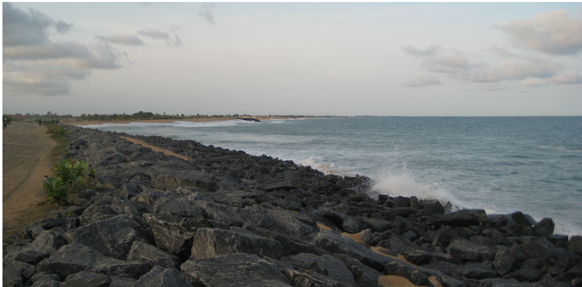
Figure 2-3: The Keta sea defence project, looking NE. In the foreground the revetment in front of Fort Prinzensten can be seen, while in the background the heads of the groynes are visible.
