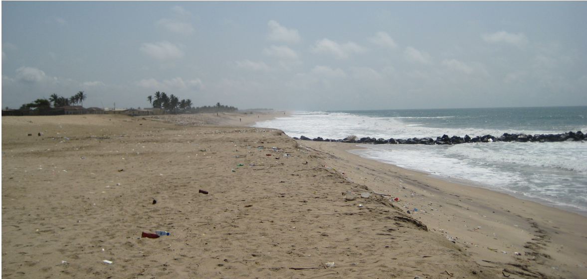
Figure 2-4: The Ada sea defence project, at Ada Foah, looking East. On the left the nourished beach barrier and to the right a groyne. The step in the coastline is an effect of the groyne partially blocking the sand.
