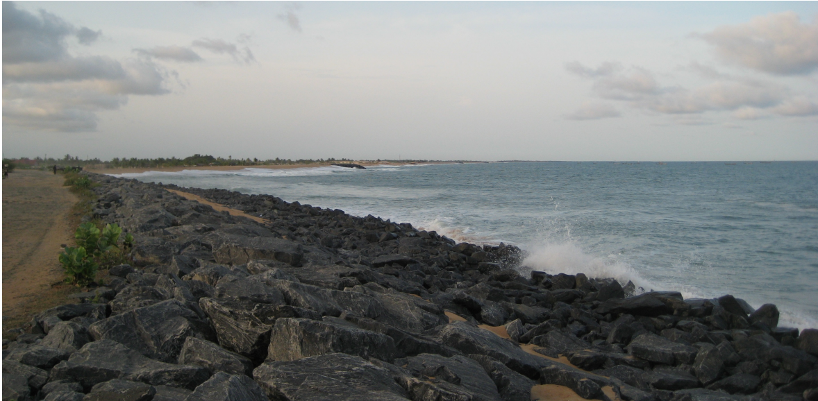
Figure 2-3: The Keta sea defence project, looking NE. In the foreground the revetment in front of Fort Prinzenten can be seen, while in the background the heads of the groynes are visible.
