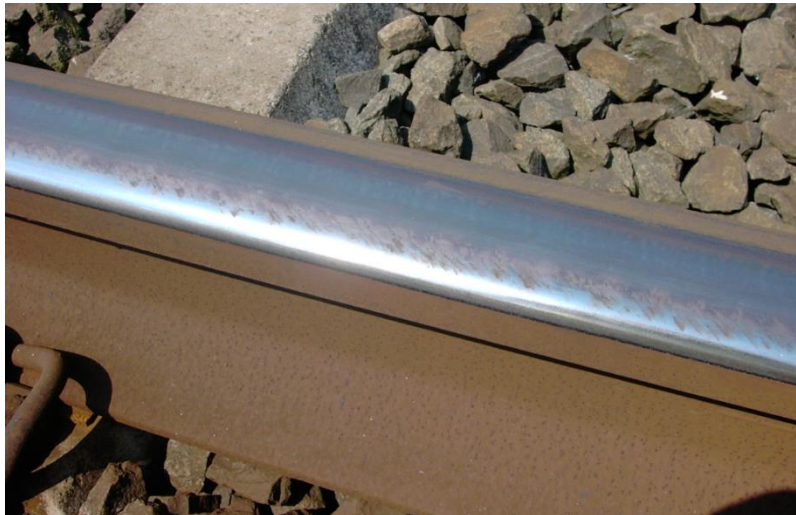
Fig. 2. High rail running surface at site A – situation prior to rail replacement (traffic direction to the right; depicted rail length about 0.36 m).
