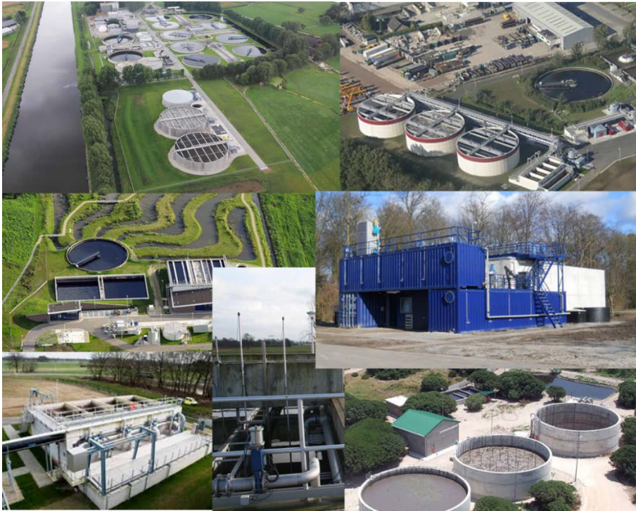
Fig. 6 - Nereda installations in Garmerwolde, Epe, Dinxperlo, Utrecht, Vroomshoop (The Netherlands) and Gansbaai (South Afrika)
