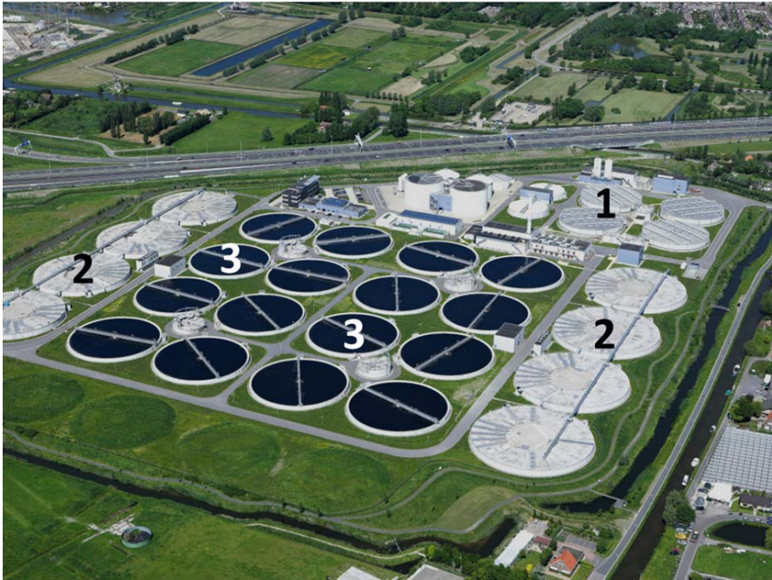
Fig. 3 - WWTP Harnaspolder (1.3 million P.E.), Den Hoorn, the Netherlands. 4x Primary clarifiers (1) 8x Secondary treatment (2) and 16x secondary clarifiers (3)
