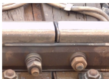
(j) IRJ number 16 with damaged insulation layer and a crack in the fastener.
