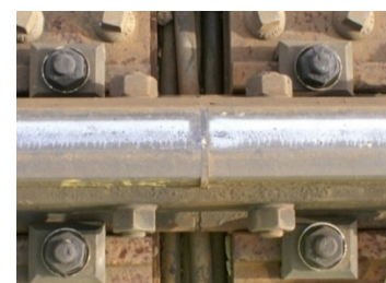
(l) IRJ number 3 on the track Groningen – Assen.
