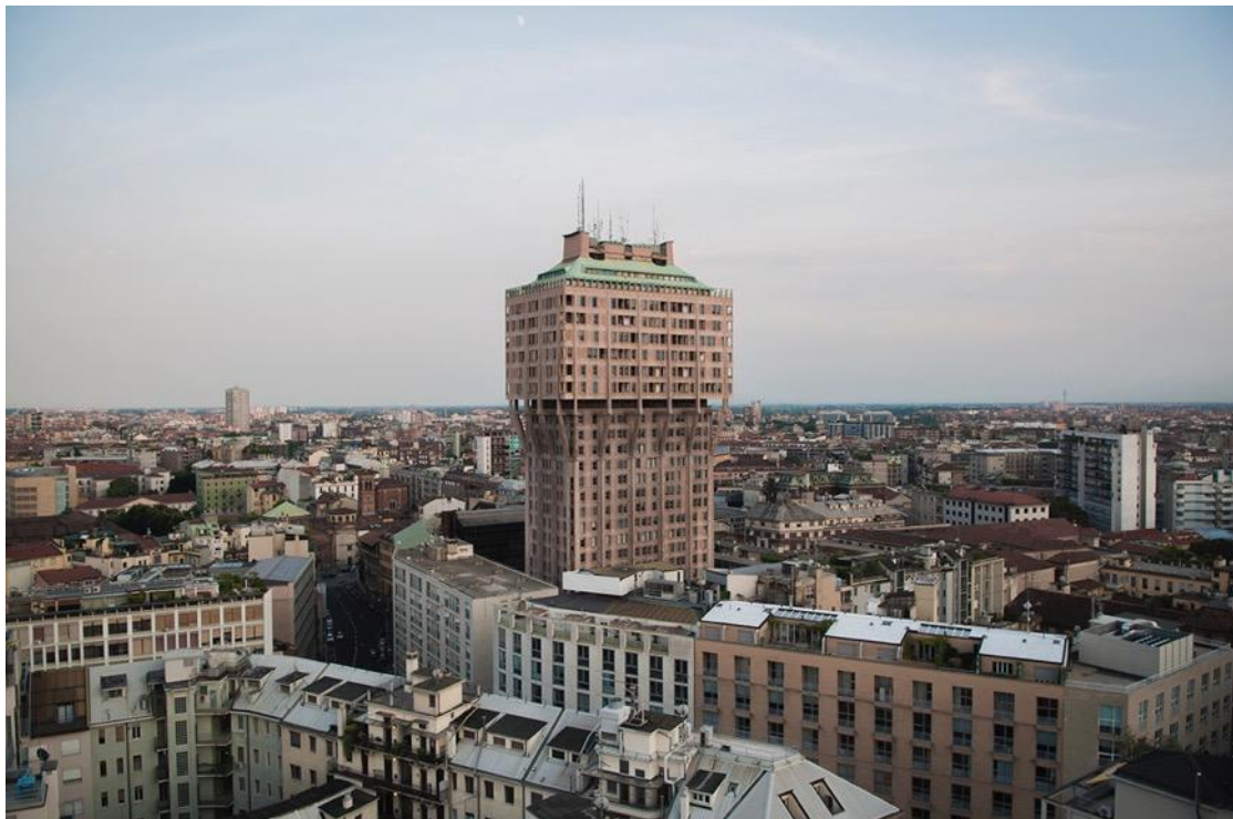
Figure 3.19. BBPR, Torre Velasca, Milan. Source: http://gbrifferraresi.tumblr.com/post/55813965468/ogni-tanto-un-po-di-torre-velasca-è-necessaria
