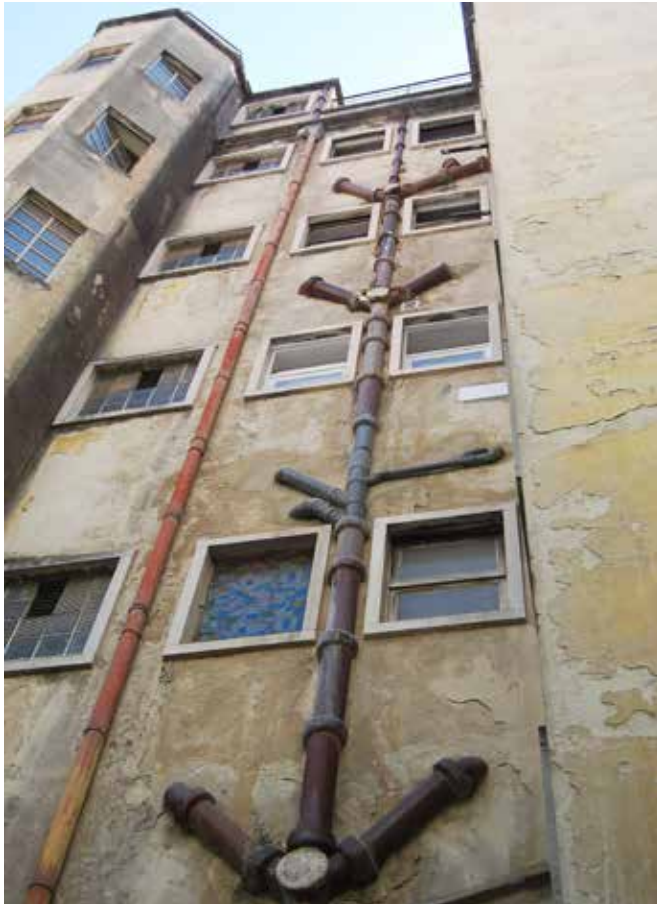
FIG. 3.39 External sewage pipes on a building in the old Carmo district of Lisbon / Marieke Kuipers
