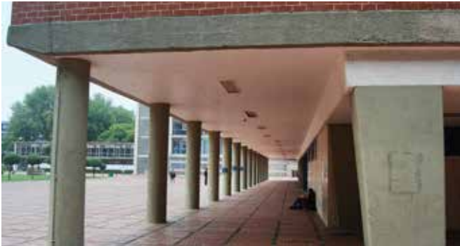
FIG. 3.22 The columns of the concrete skeleton structure exposed on the ground floor level of one of the National University campus buildings (UNAM) of Mexico; the layout of the campus' pavement is also part of a structured design / Marieke Kuipers
