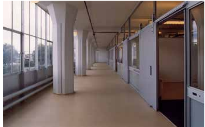
FIG. 5.28 A view inside the double-skin façade at the eastern side, where the cavity doubles as a corridor, required for proper circulation in any case / Fas Keuzenkamp, Pijnacker
