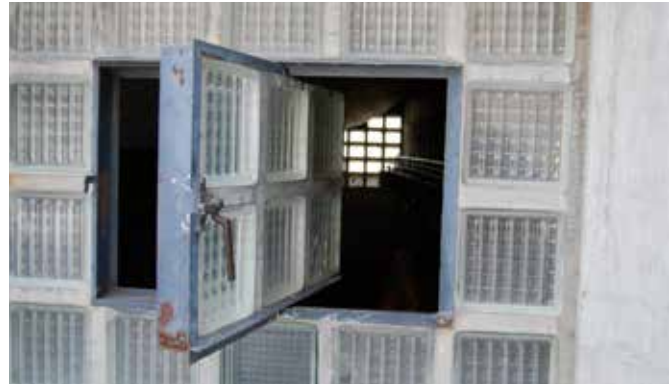
FIG. 4.10 A typical detail of modern heritage: a steel framed window with traces of corrosion in a wall of glass bricks, part of the Salime Hydro Power Plant / Marieke Kuipers
