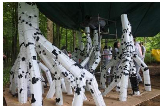
Figure 8. Polypropylene form-work with steel reinforcement bars on site.
