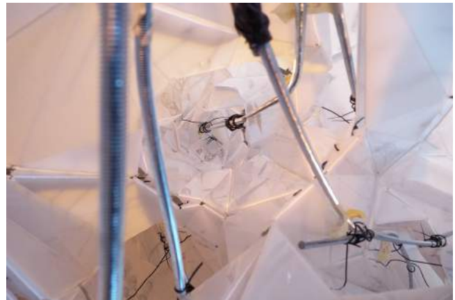
Figure 7. Steel rod reinforcement bars placed inside Polypropylene form-work.
