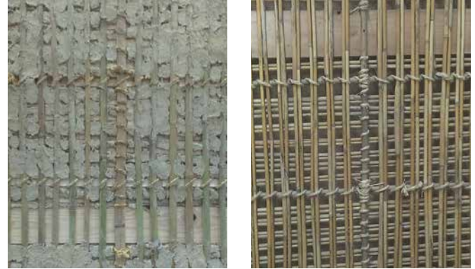
FIG. 4 Wooden frame with bamboo lattice bound by rice ropes on which the first, inner layer, of the earth wall has been applied (left). Wooden frame with reed lattice, before the application of the earth plaster (right)
