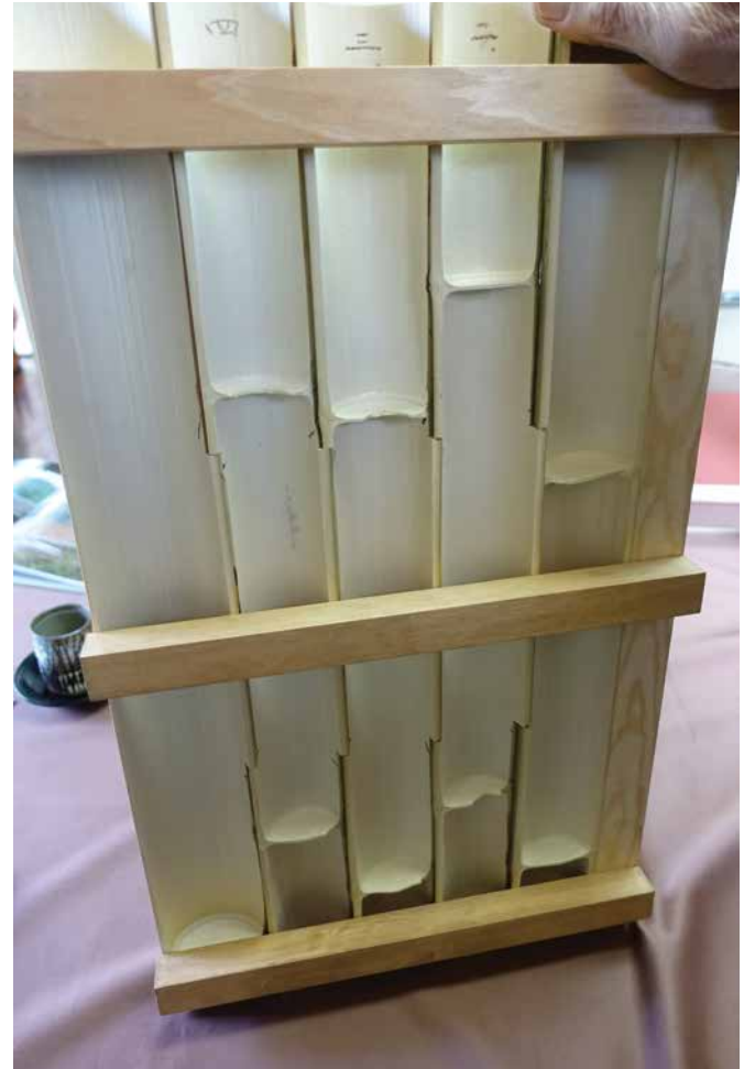
FIG. 27 The back reveals the cuts and adjustments necessary to give the front its regular appearance. In the office of Yoshiaki Namakura of Sotoji construction
