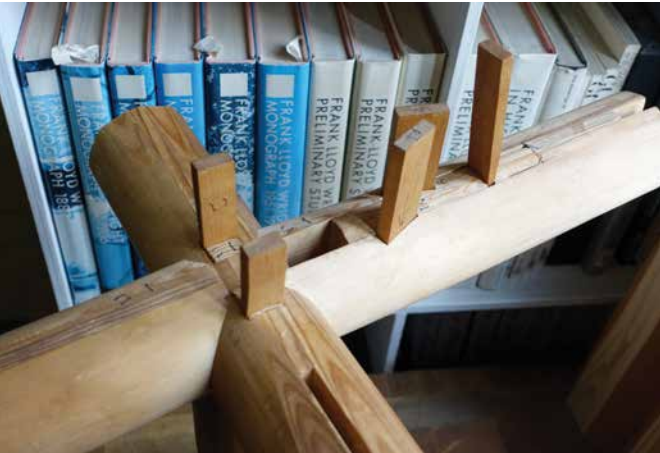
FIG. 10 Detail of post and beam
