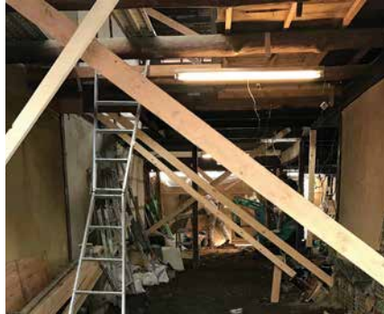
FIG. 4 Machiya under renovation
