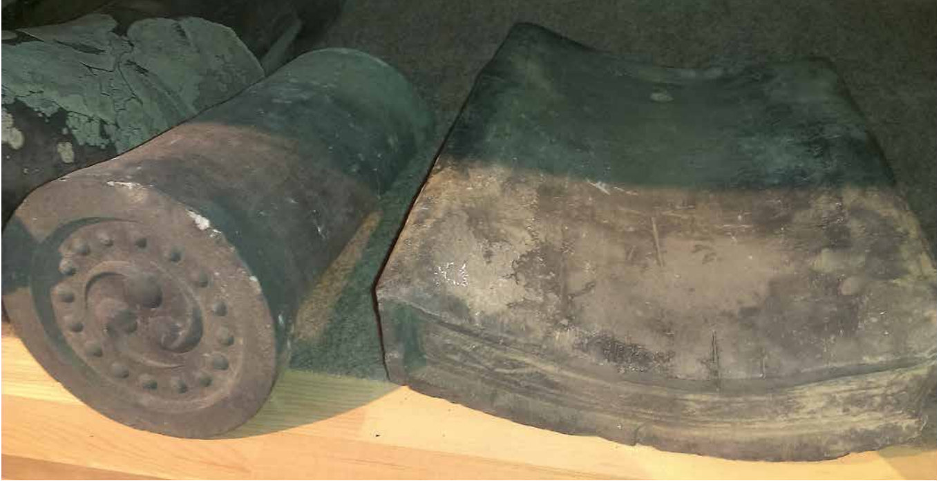
FIG. 18 The interlocking system used in ancient Japanese tiles
