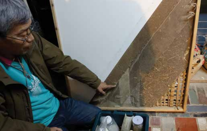
FIG. 20 Hiroyuki Sato explains the seven layers of plaster work
