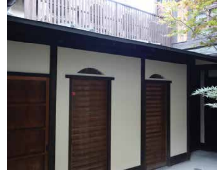
FIG. 8 Additional building of Kamanzacho-Choie
