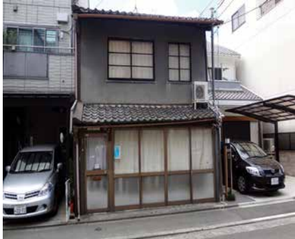
FIG. 3 Machiya before renovation
