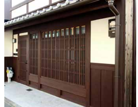
FIG. 5 Machiya after renovation
