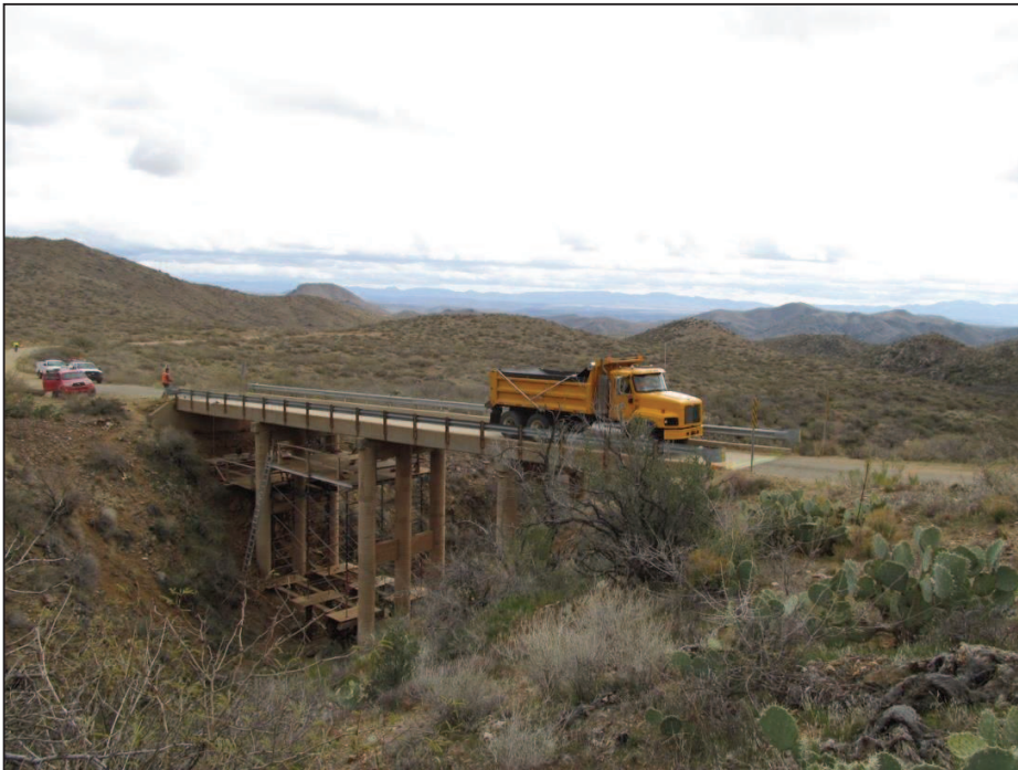
9 10 Figure 1. Diagnostic load test on a rural one-lane concrete slab bridge 11 Diagnostic load testing has gradually gained wider acceptance among bridge owners as a 12 refined method for bridge load rating, especially when simplified analytical methods suggest
