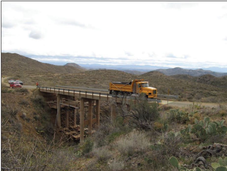
9 10 Figure 1. Diagnostic load test on a rural one-lane concrete slab bridge
