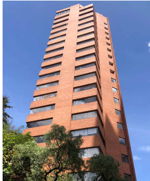
FIG. 5 Building of the Colombian Society of Architects by Rogelio Salmona and Luis Torres, 1974. (Photograph by Faculty of Architecture & Design, Universidad de los Andes)
