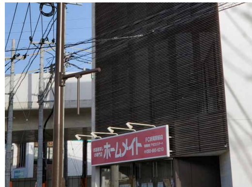
FIG. 4 Horizontal koshi in a commercial building in Kitakyushu, Fukuoka
