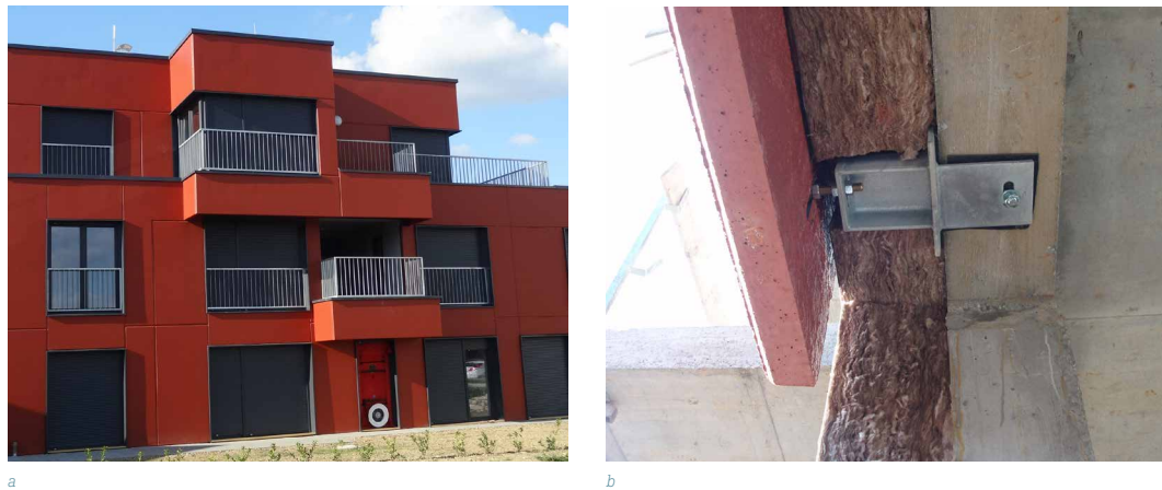
FIG. 10 “First ECO-SANDWICH® house”: a) south façade; b) thermal break for anchoring systems
