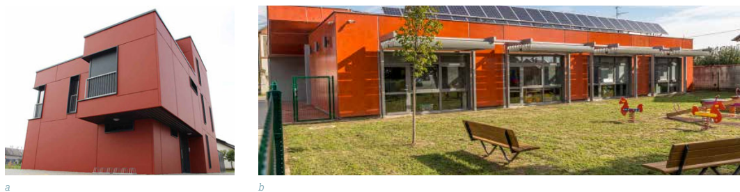
FIG. 9 First implementation of prefabricated modular façade panel from RAC: a) family house "First ECO-SANDWICH® house"; b) kindergarten "Ribica" (Cist racun, 2017)
