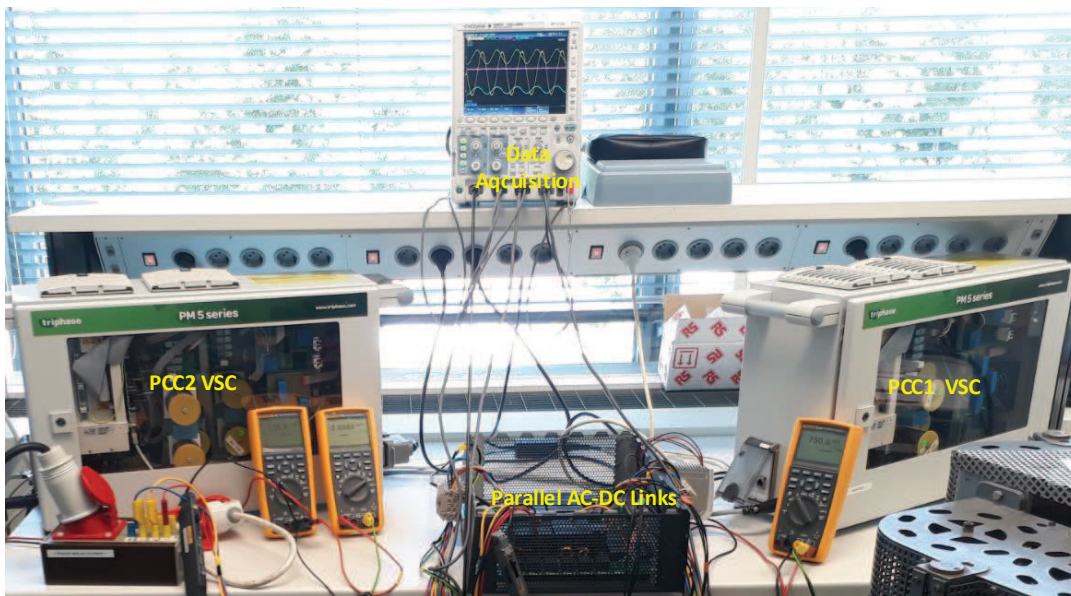
Fig. 11: Experimental set-up to study the CMC in parallel operating ac and dc links.
