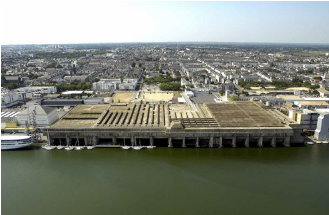
FIG. 5.7 The aerial image of the roof
