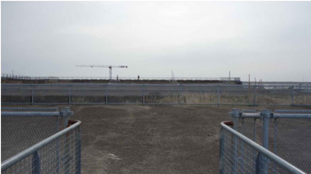
FIG. 5.23 Layers of fences on the roof
