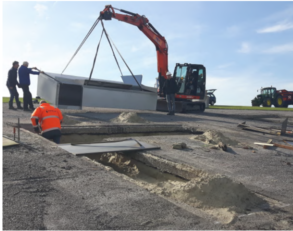
Figure 7.3: Excavation of the dike slope and placement of the overtopping tanks inside the dike.
