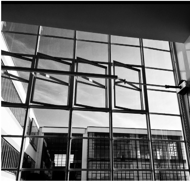
FIG. 5.8 Bauhaus Dessau, staircase, office and workshop glazings were originally using polished plate glass to achieve a precise and industrial look / Photo: pixy.org
