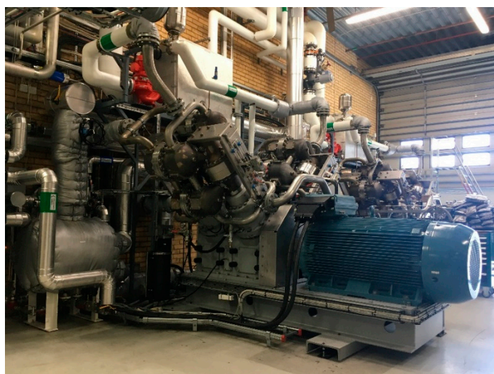
Figure 2. The highlift Stirling-cycle-based heat pump (SC HP) developed by Olvondo Technology, Norway and being used by the pharmaceutical company AstraZeneca, Gothenburg, Sweden.
