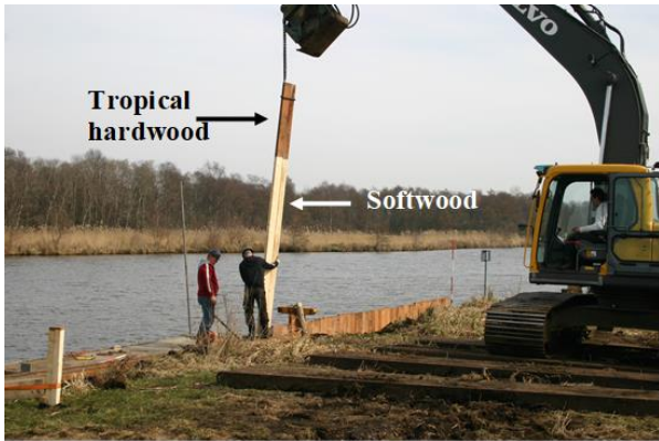
Figure 1: Twin-wood sheet pile, (Taken from FORECO houtproducten., https://www.foreco.nl/nl/producten/twinwood ).
