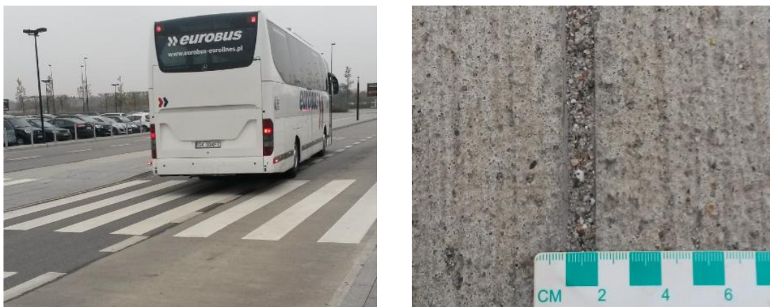
Fig. 7.3.3. Sealed joints contaminated with incompressible material at bus stop, Wroclaw city, Poland.
