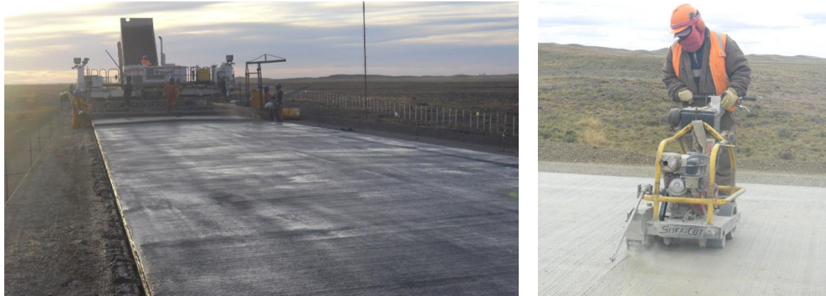
Fig. 5.5.2. Paving with slipformer (left) and (early-entry) saw-cutting of the transverse joints (right)
