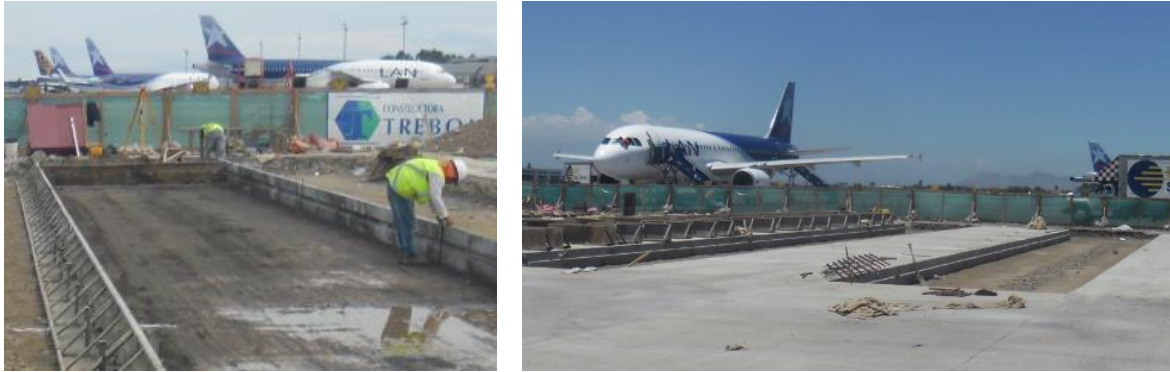
Fig. 5.5.4. Paving with fixed formwork (left) and general view of the test section (right).
