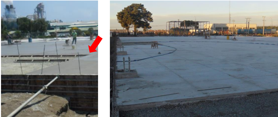
Fig. 5.5.3. Construction of industrial floor with shorter irregular sections (left) and general view of the industrial floor (right)
