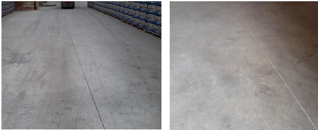
Fig. 7.3.11. General view of the industrial floor and an example of joint state (Pradena & Diaz, 2016)
