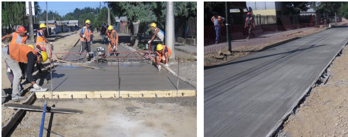
Fig. 5.5.1. Paving with fixed formwork (left) and general view of the test section (right).
