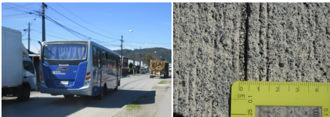
Fig. 7.3.5. Traffic and UnJs state in JPCP in a street in an ultra-high rainfall zone (saw-cut 3 mm) (Pradena & Houben, 2015a).
