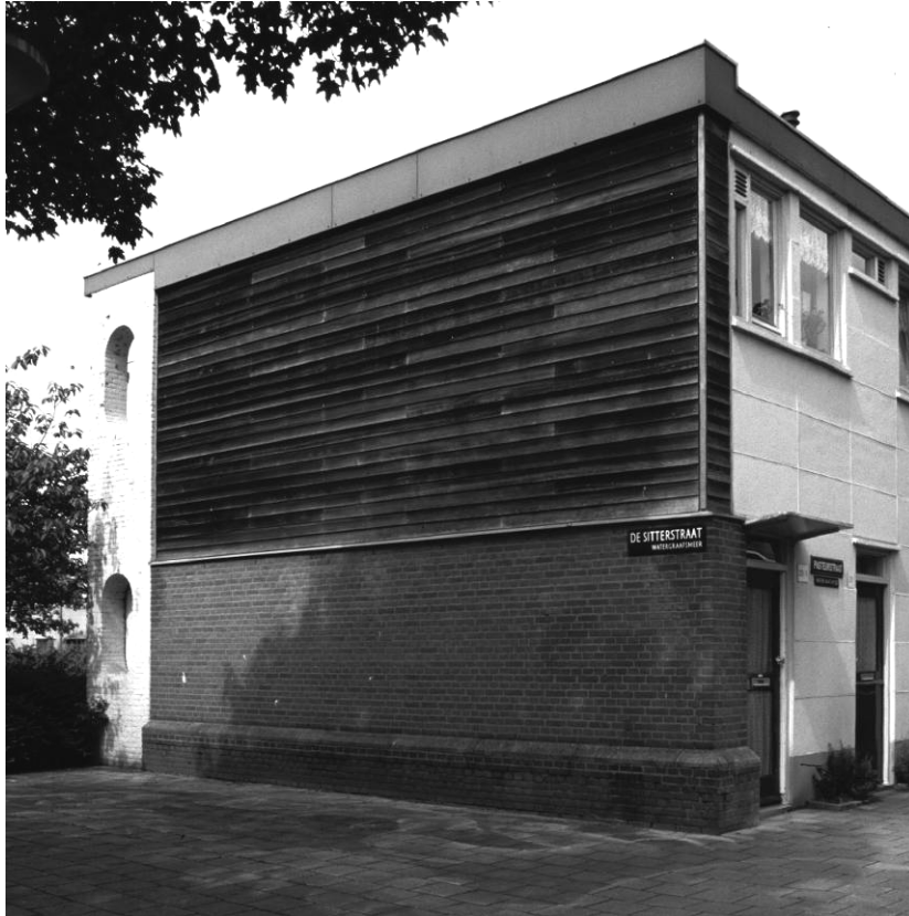
Figure 13: facade covered with wood and brick around 1987.
