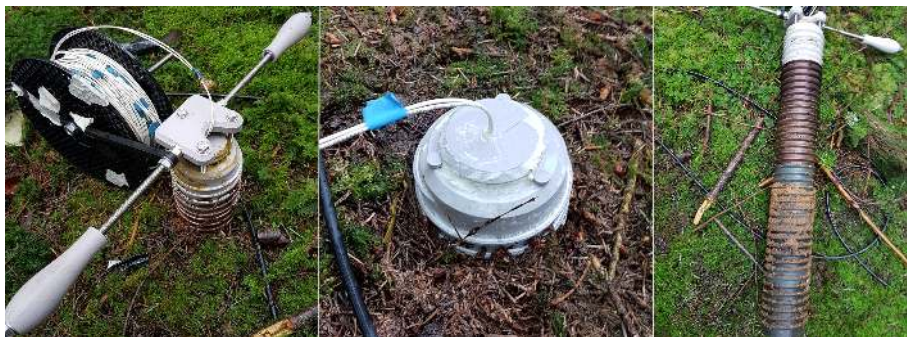
Figure 7.3: Installing the DTS probe using the installation tool (left), the probe during installation (center), and the probe after removal (right).
