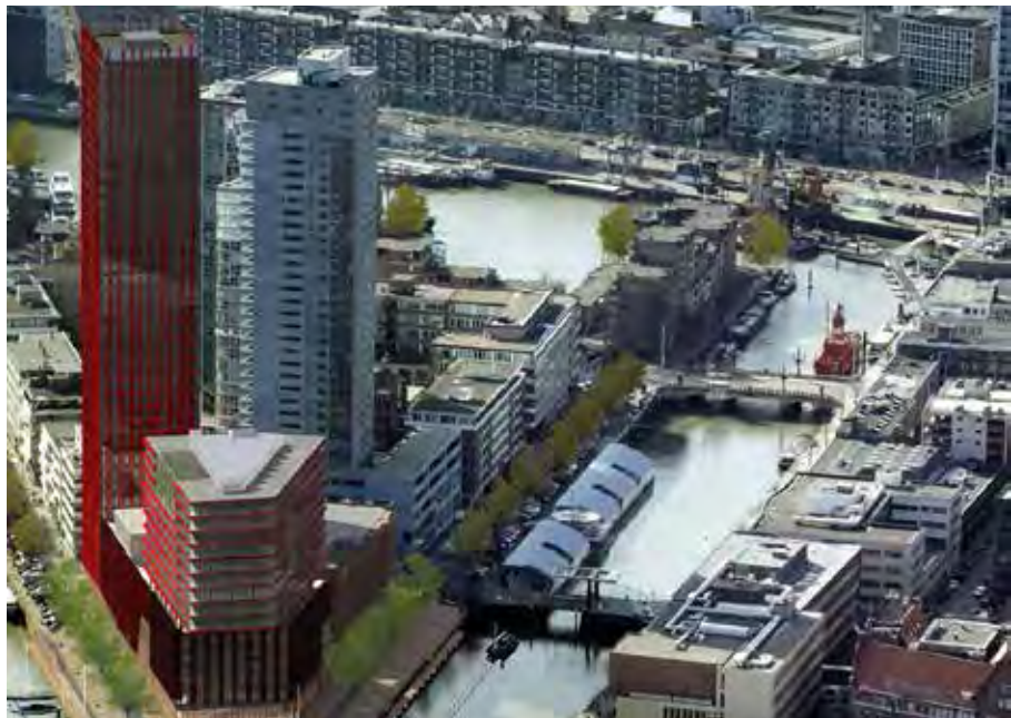
Figure 12 Towers of Wijnhaven Island in development.
