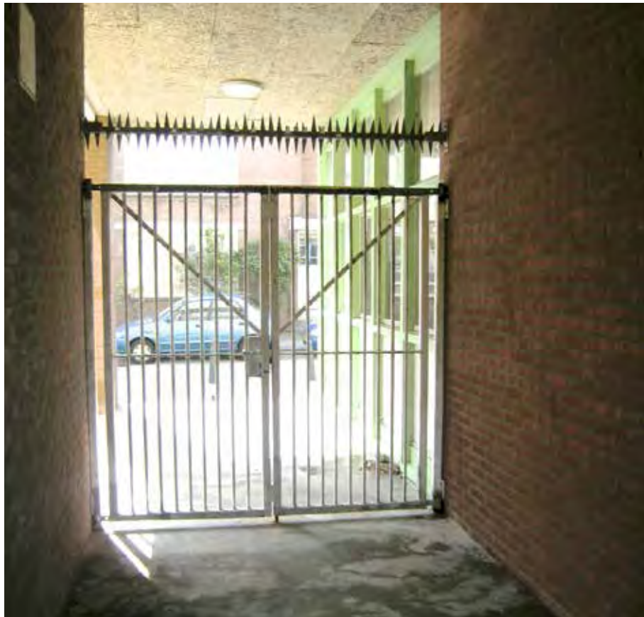
Figure 84 A locked courtyard gate in Oude Westen.
