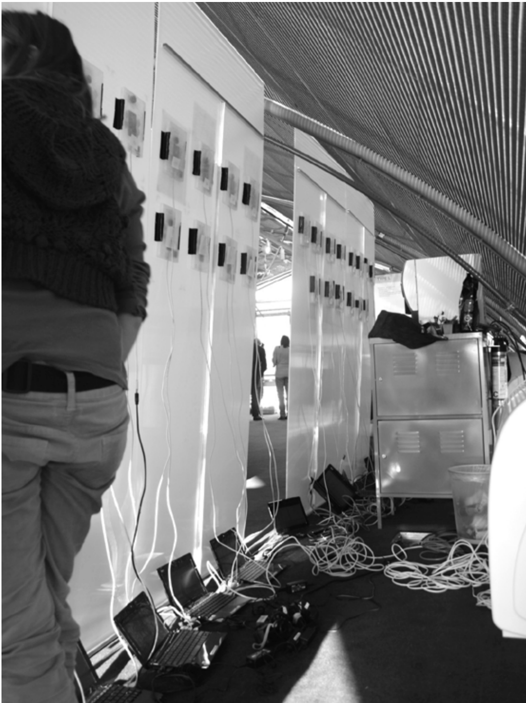
Figure 126 The technical equipment behind the voting station.
