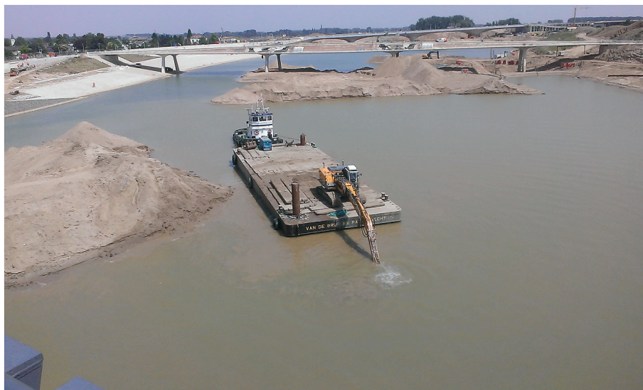
Fig. 7. Excavation of floodway at Nijmegen (July 2015).
