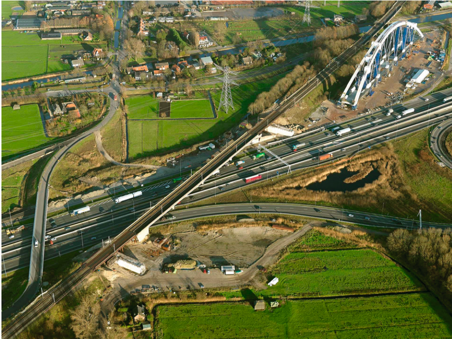
Figure 4.4: Spoorbrug Muiderberg Bridge during construction (current name: Zandhazenbrug) (source: Rijkswaterstaat)
