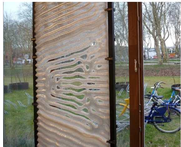
Fig. 13 – Installed full panel of the prototype of the developed PCM based Trombe wall in a meeting room.
