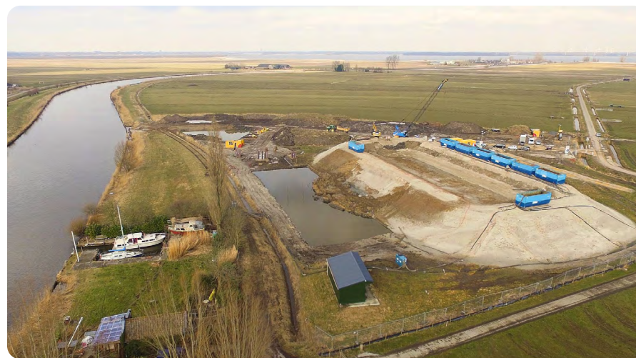
Figure 1: The full-scale Eerdijk test site from an aerial perspective. Photo © NOS / Eric Feijten.
