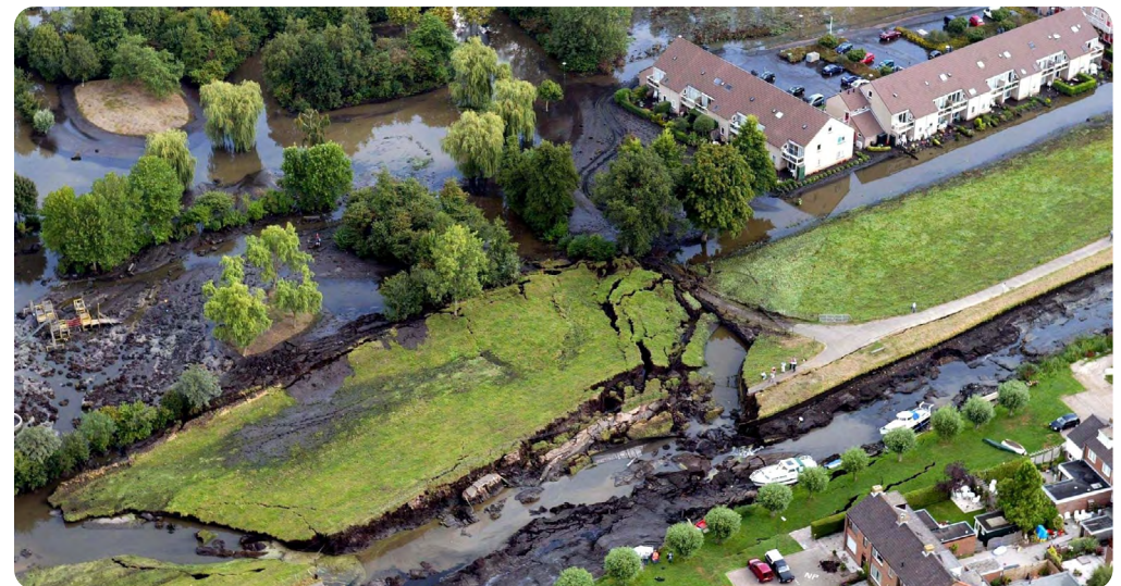
A sudden horizontal dike slide in August 2003 due to a hole of 60 metres in the dike flooded Wilnis. Photo © ANP.
