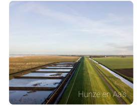
3 Wide Green Dike
