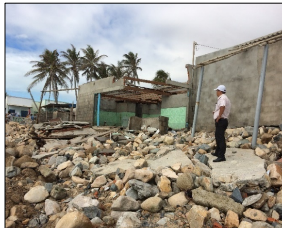
b. Protection after damage and sliding.
