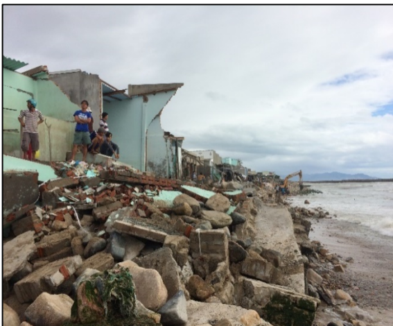
a. Houses are damaged by erosion.
