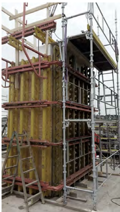
Figure 4.3: Onsite prefabrication using a standard, rectangular scaffolding for formwork support against bespoke EPS infills.
