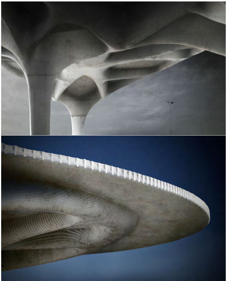
Figure 3.18: top The Unikabeton Project bottom Structure from the milling process
