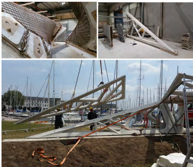
Figure 3.32: Reinforcement of element B1 (top, left) and element A1 after casting (top, right). Bottom: assembly of element A1 on A2, B1–B2
