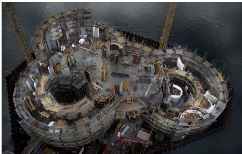
Figure 4.2: Construction site overview: the robotically hot-wire-cut formwork is used in combination with standardised timber and steel modules to resist casting pressure, applied for creating the hyperbolic void openings of the cylindrical main walls Photo: Kirk Property A/S.
