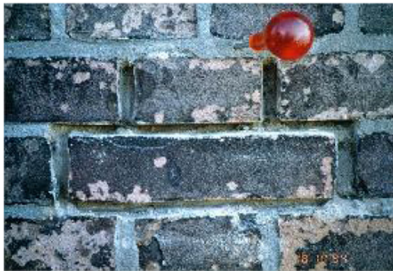
Fig. 18 Weak, decayed trass lime re-pointing
