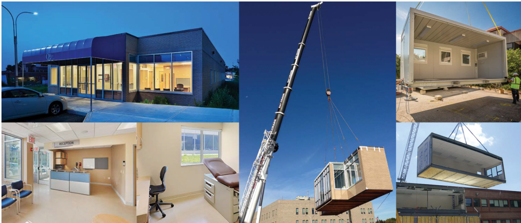
FIG. 4.32 Modular construction in hospitals example [342]
