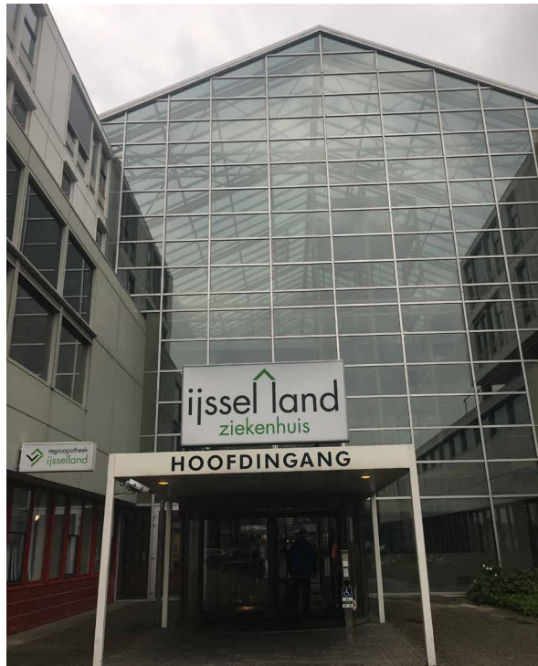
FIG. 3.26 Hospital main entrance
