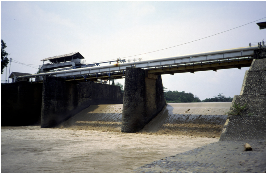
Figure 5.2 The modern weir Salamderma
