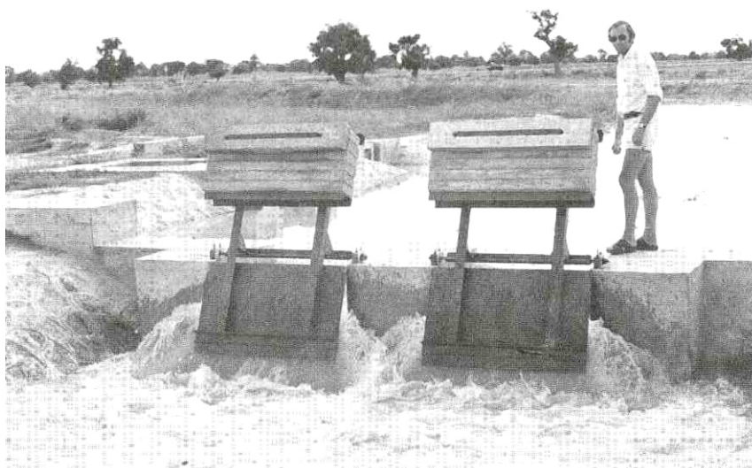
Figure 7.10 Begemann automatic gate in the Kano River system, Nigeria 90
