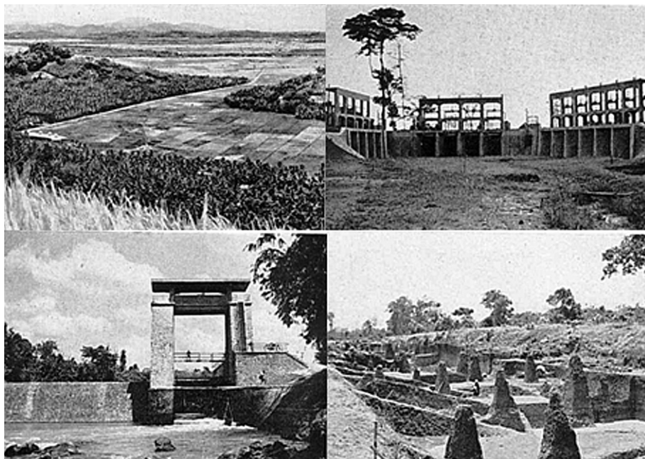
Figure 7.4 Impressions from the Way Sekampung area 58 Top: Left: Irrigated sawahs; Right: Trimurdjo distribution structure. Bottom: Left: Argogoeroeh weir; Right: Construction of main canal
