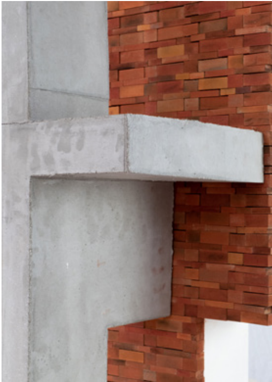
Fig. 11.6 Concrete and MDF model of the meeting of two walls from different times, scale 1:5, Riccardo Garrone and Sam Stalker, detail. Photograph: Bas Leemans.
