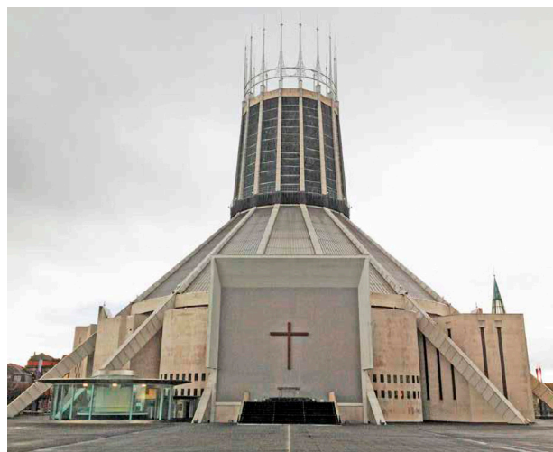
Figure 1. The dalle de verre lantern crowning Liverpool Metropolitan Cathedral, viewed from the north. Courtesy of Purcell UK
