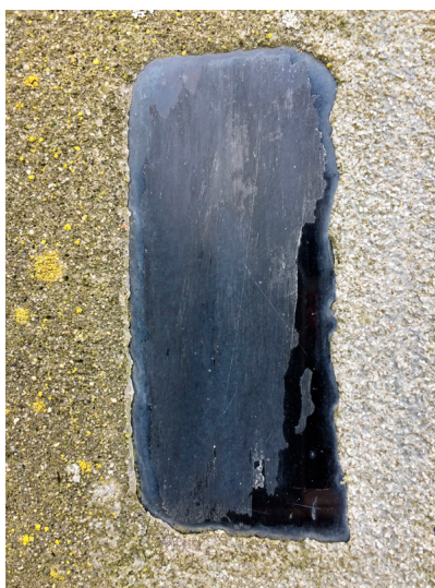
Figure 4. Weathering of the 1990s polymer coating on the exterior of one dalle de verre slab. Courtesy of Norman Tennent
