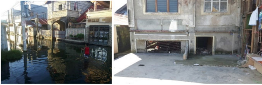
Fig. 2 Flooded streets and ground subsidence in the Pampanga delta
