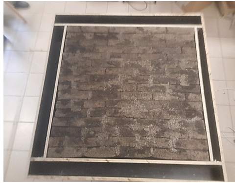
Fig. 10. side enclosure with wooden frame.
