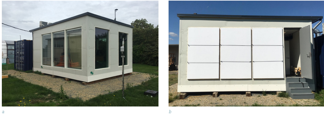
FIG. 2 Exterior views of MATELab: a. View of the south-west building envelope; b. View of the east building envelope with cover panels.
