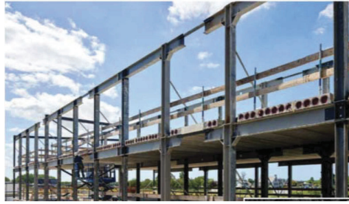
Figure 3. Construction of Biopartner 5, whereby steel elements are used from the neighboring Gorlaeus-building (Terwel et al. 2021).
