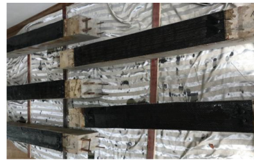
(c) Finished RC beams reinforcement.
